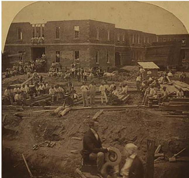
New PA Hospital for the Insane being built in 1859
